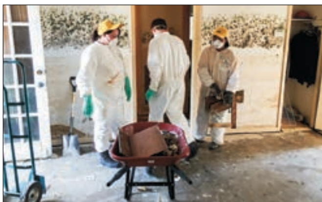
▲ Protective clothing and gear was necessary in toxic conditions following Hurricane Harvey.
