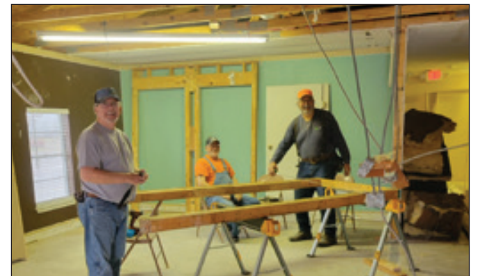
▲ The Master's Builders working at Anthony Drive, Ennis
