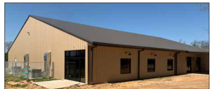
▲ New fellowship building, currently under construction
